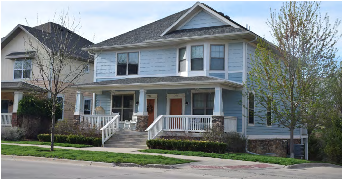
Example of a Porch
