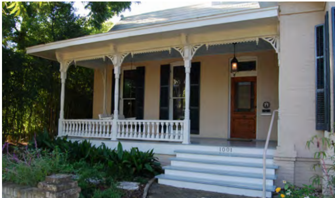
Example of a Porch
