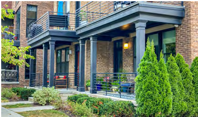
Example of a Porch
